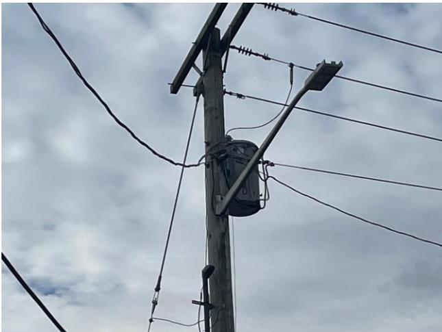
Closer view of the transformer. No markers could be observed. There was no evidence of leakage or staining observed on the transformer, pole and surrounding sidewalk.
