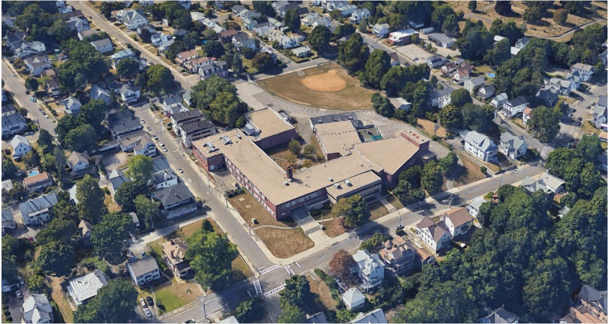
The existing AMS Middle School located at 115 Howard Avenue
