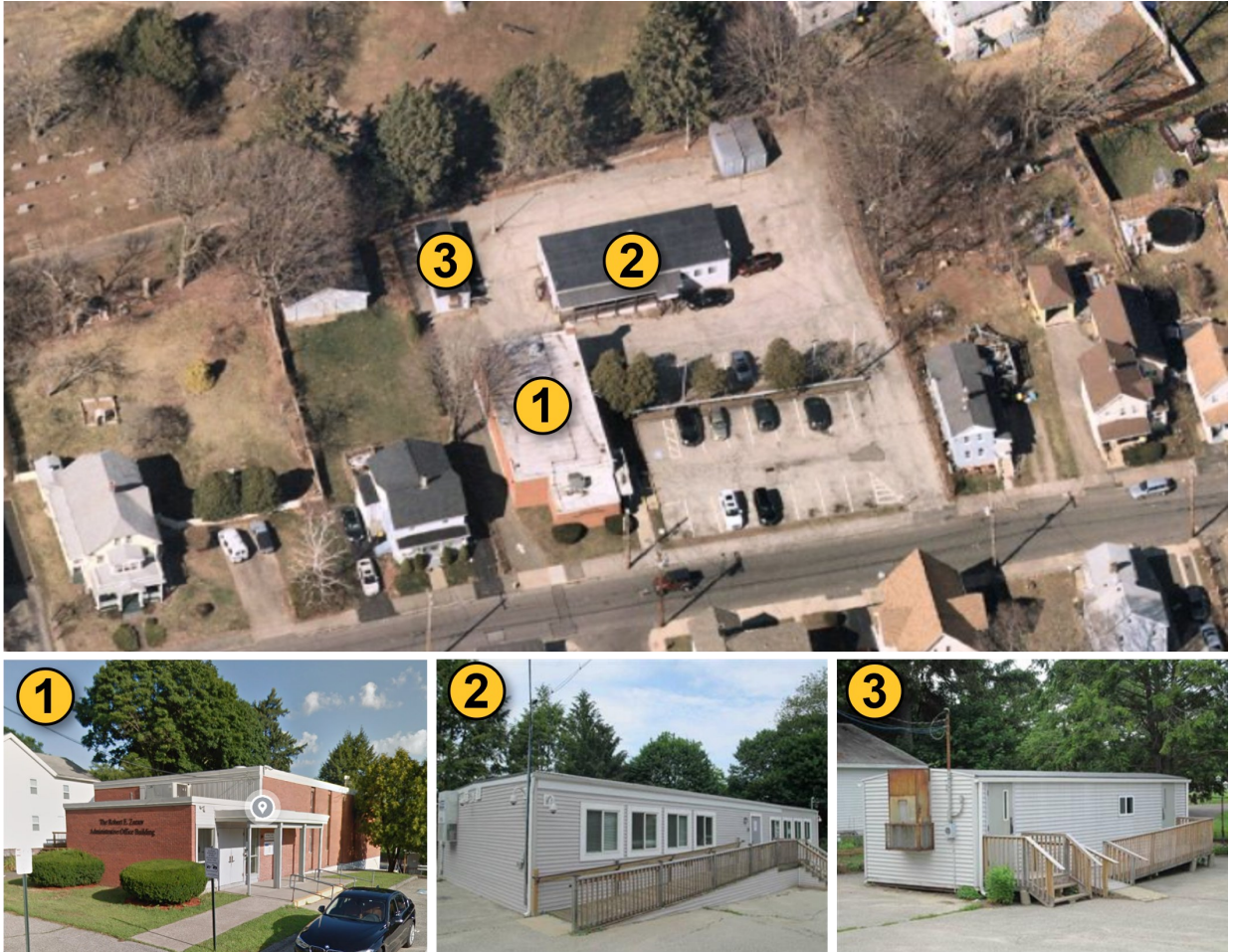
The existing Central Office space located at 42 Grove Street. The site consists of the main building (1), modular building (2), and trailer (3).
